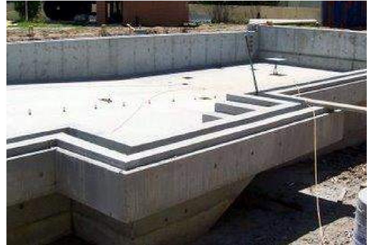
Figure 6.2: In-situ Reinforced Pool Tank Design at Grade
